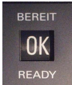
Ready to Close Indication Unique to Siemens 3WL
